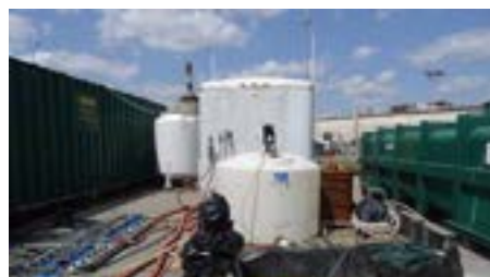
LNAPL SEAR Project: Injection of 260,000 gallons TASK™ ASB/polymer formulation, followed by 780,000 gallons of water, and recovery of same with LNAPL.
